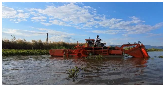
Figure 3. Rehabilitation Activities Conducted Following the 2024 Flood and 2025 Earthquake (Hyacinth Removal and Dredging Activities)
