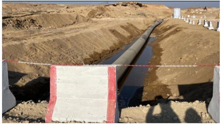
Figure 4 Typical pipeline open trench excavation
