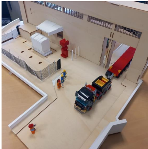
Model of a powerhouse to prepare the change of transformer
