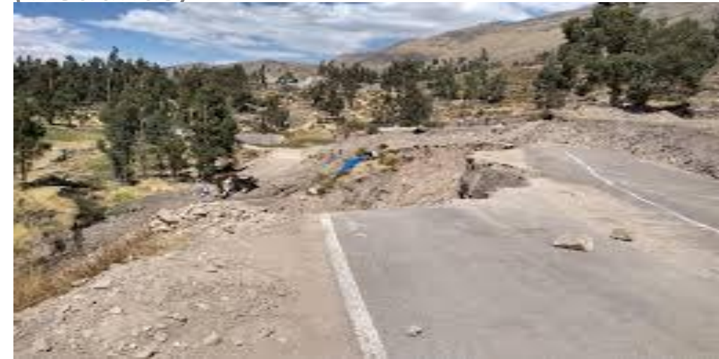
Geological Instability, recurrent landslides in Maca district
