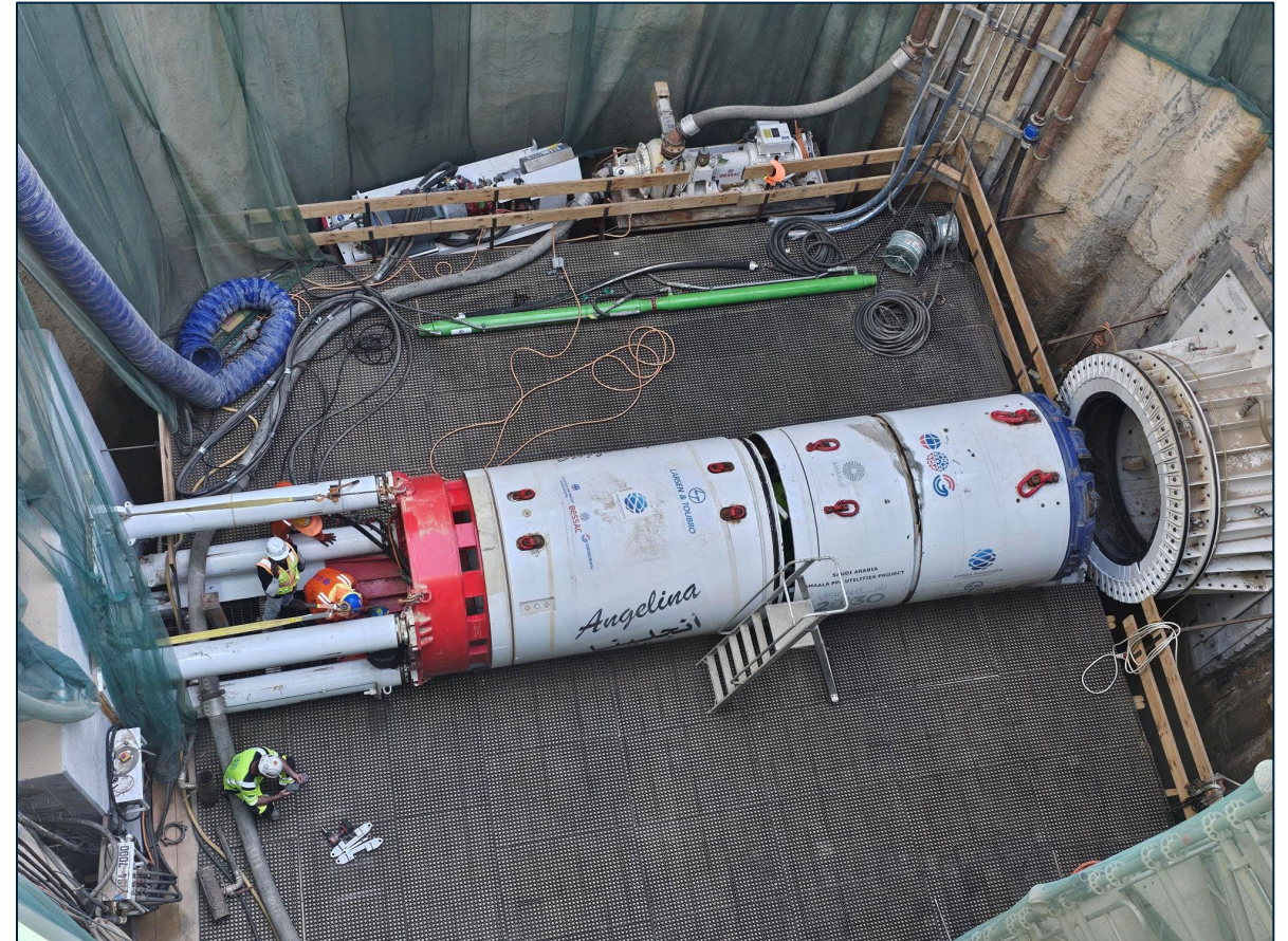
Photograph of Micro-Tunnelling Machine inside the RO Plant Outfall Shaft
