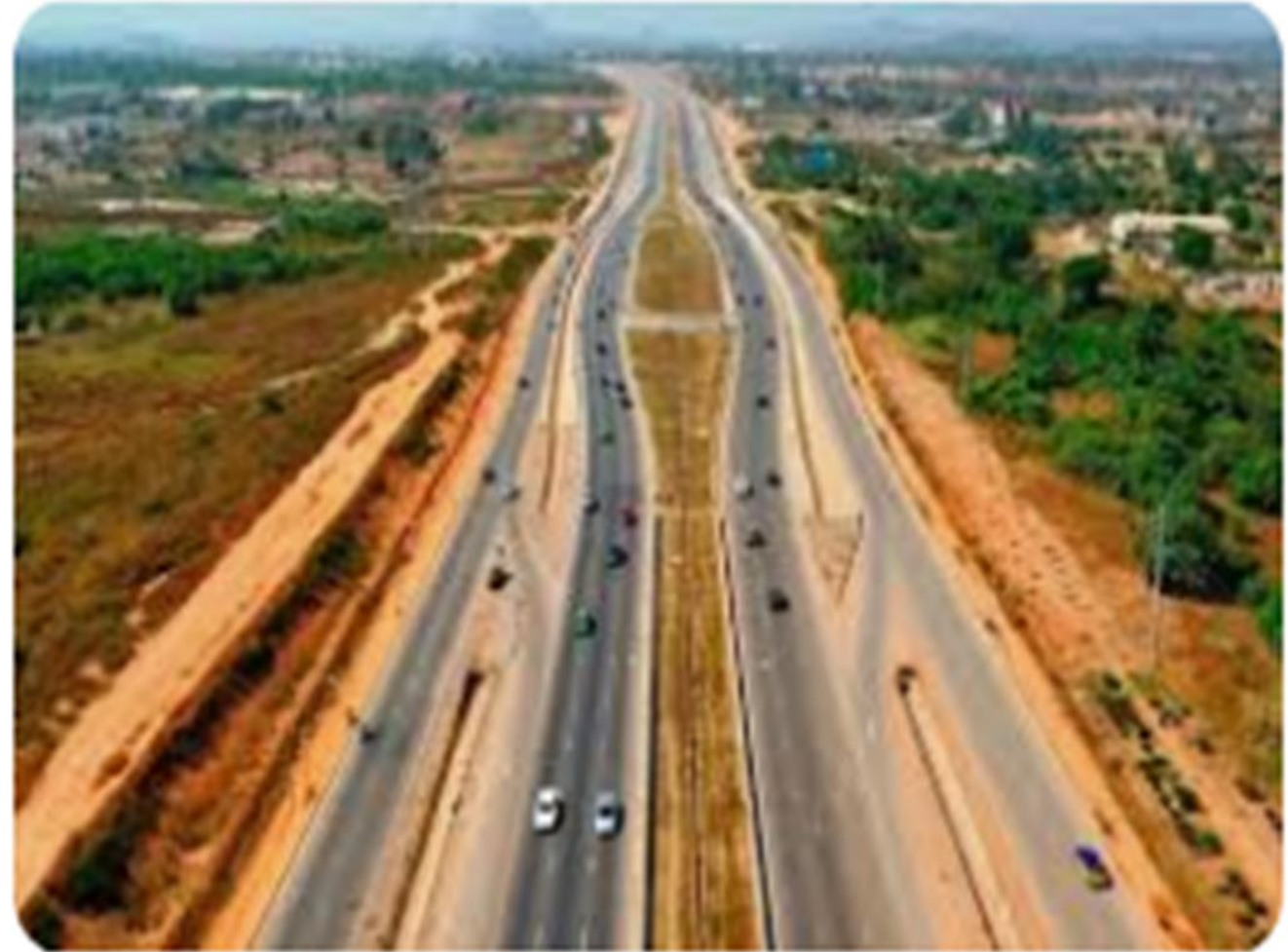
Fig 3 The Road Construction
